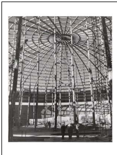
Left: Roof with no panels
