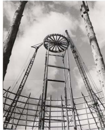
Above: Installing Center Ring
